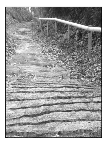
As can be seen from the photos a solid hand rail has been erected and the very slippery part has been corrugated making it safe in wet weather.
